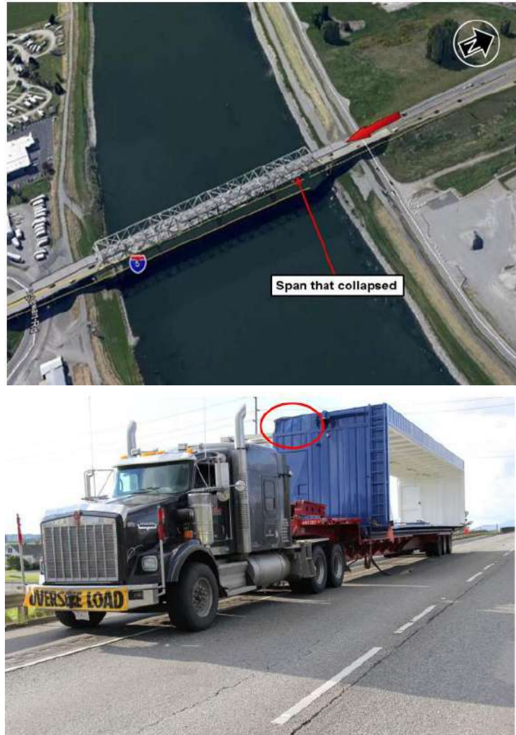
Figure 5-3: Collapse of the Interstate 5 Skagit River Bridge
