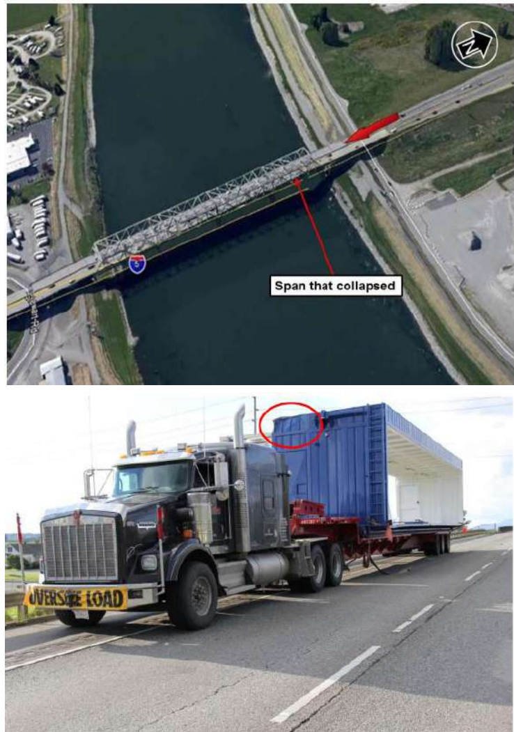
Figure 5-3: Collapse of the Interstate 5 Skagit River Bridge
