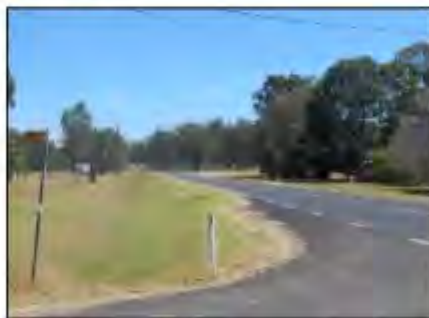
Figure 5 Tumoulin Road / Condon Road - Looking North
