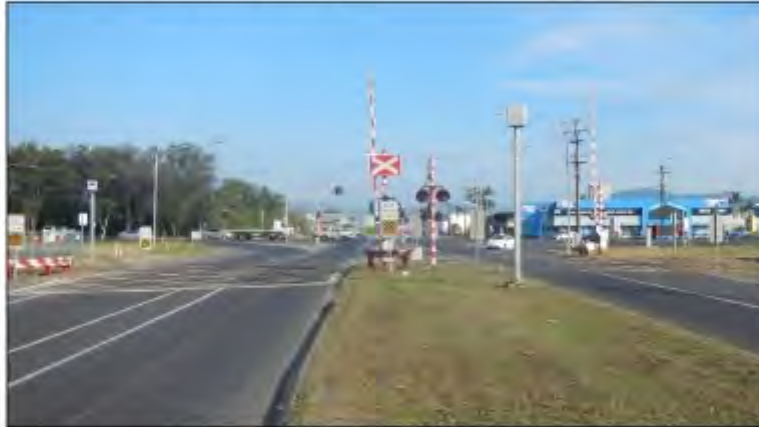
Figure 14 Rail Level Crossing (North Coast Line) – Aumuller Street, Calms
