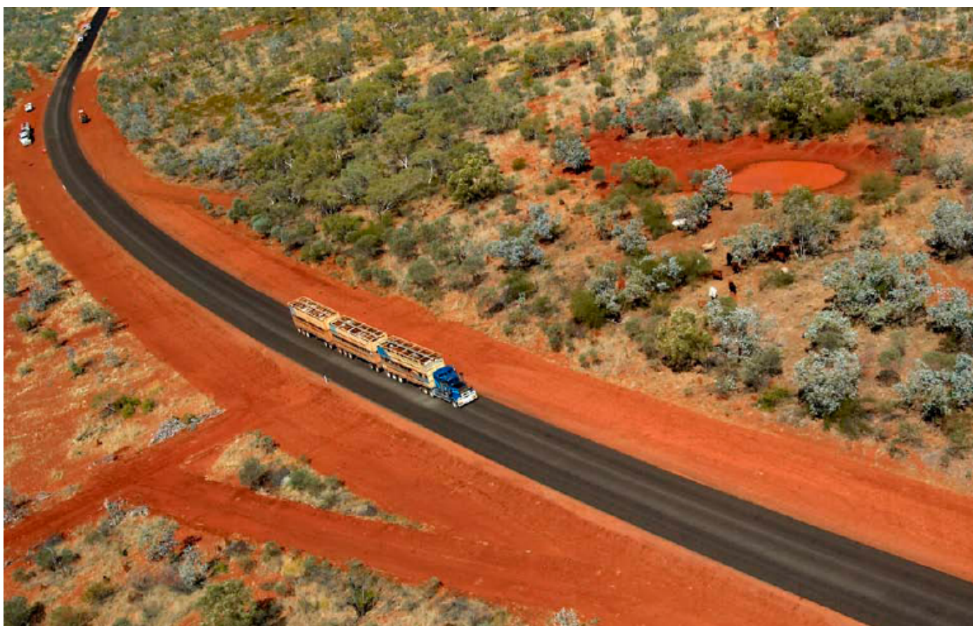
Figure 7.10: NEWLY SEALED DEVELOPMENT ROAD
